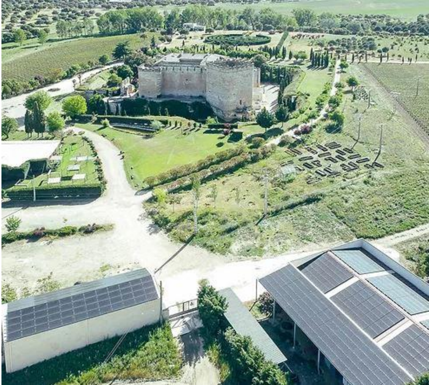
Solar panels on the roof of auxiliary and contemporary buildings near a Listed Castle (Spain)
